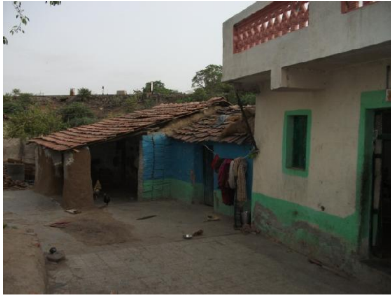
Figure 7: House extension given out on rent
